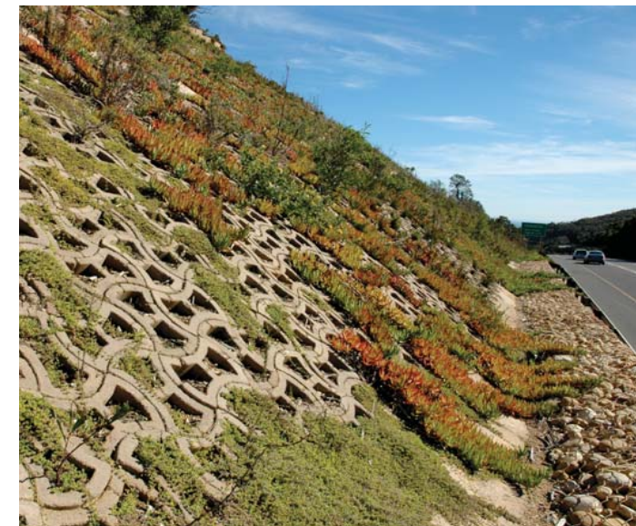
23064 blocks were used to stabilise this slope
