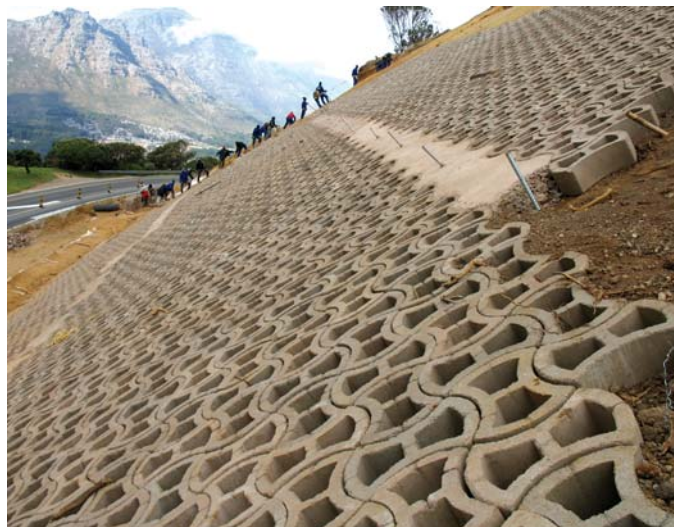
23064 blocks were used to stabilise this slope
