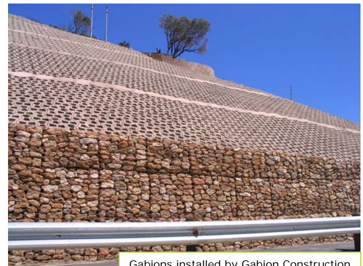
Gabions installed by Gabion Construction
