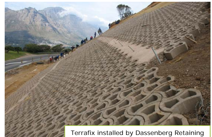
Terrafix installed by Dassenberg Retaining
