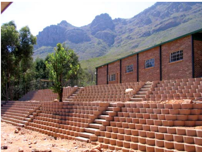
Terraforce and 4 x 4 multi stairs installed by Dec 2005
