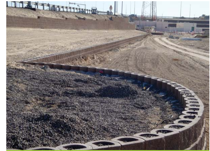
Landscaping features with L16 Terraforce blocks
