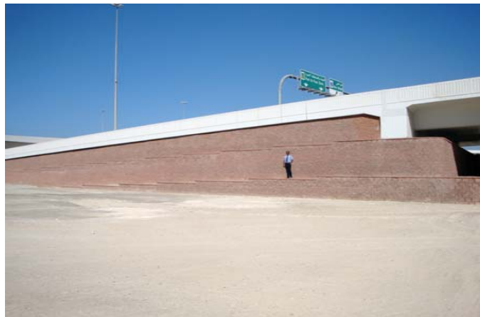
Jebel Ali Interchange Dubai. Terraforce L16, Consent LLC
