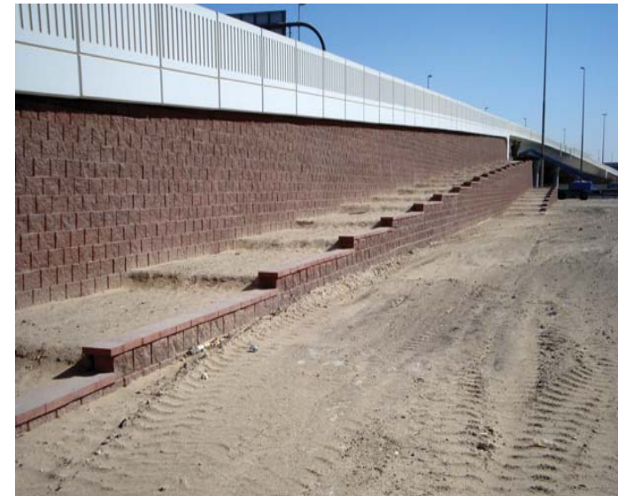
Landscaping steps and concrete capping.
