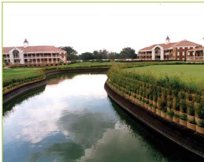
STORM WATER COLLECTION PONDS
