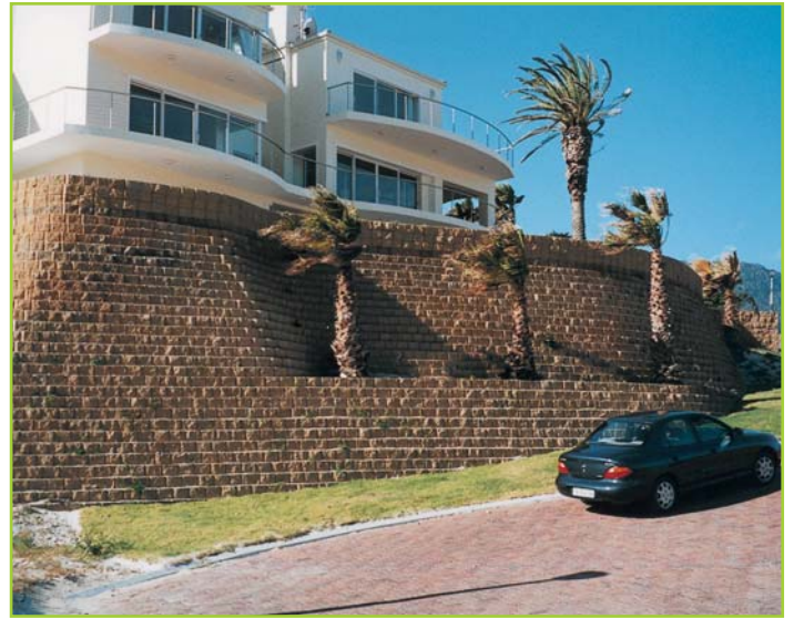
COMPOSITE WALLS IN SPLIT FACE FINISH
